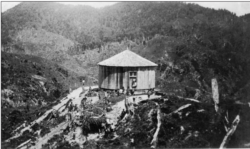
Figure 4: The whare kanikani, described as 30ft in diameter with walls 11½ feet high, in use as a school house c.1921. In front is a mud slide made by the students. Photographer unknown, Alexander Turnbull Library, Wellington, F-30908-1/2.
